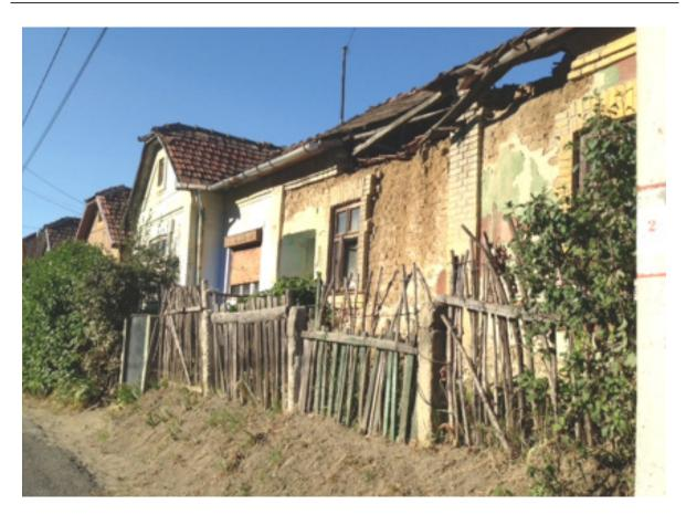
Figure 4. Architectural, public health and epidemiological state of the dwellings were unacceptable. Buildings leaked, the walls were damp and mouldy. Hygienic facilities (running water, bathroom), proper ventilation and modern heating possibilities were all lacking. Dogs and cats were also kept in some of the dwellings thereby increasing possible risk of infections.
